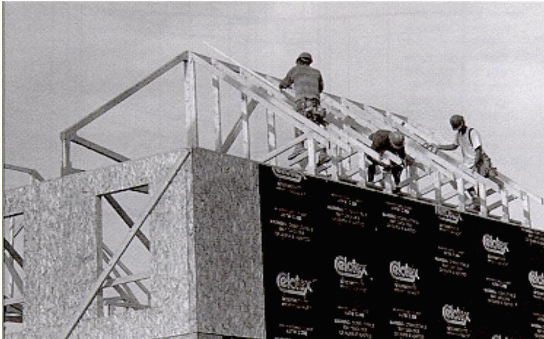
This worker has installed a slide guard on this 8:12 pitch roof eave. The slide guard is a roof bracket with a 2x6 at a 90 degree angle. In this case, the worker is wearing-although not required-a safety belt and lanyard to prevent a fall. After the shingles are placed beyond 8 feet of a roof line, more slide guards will be installed.
