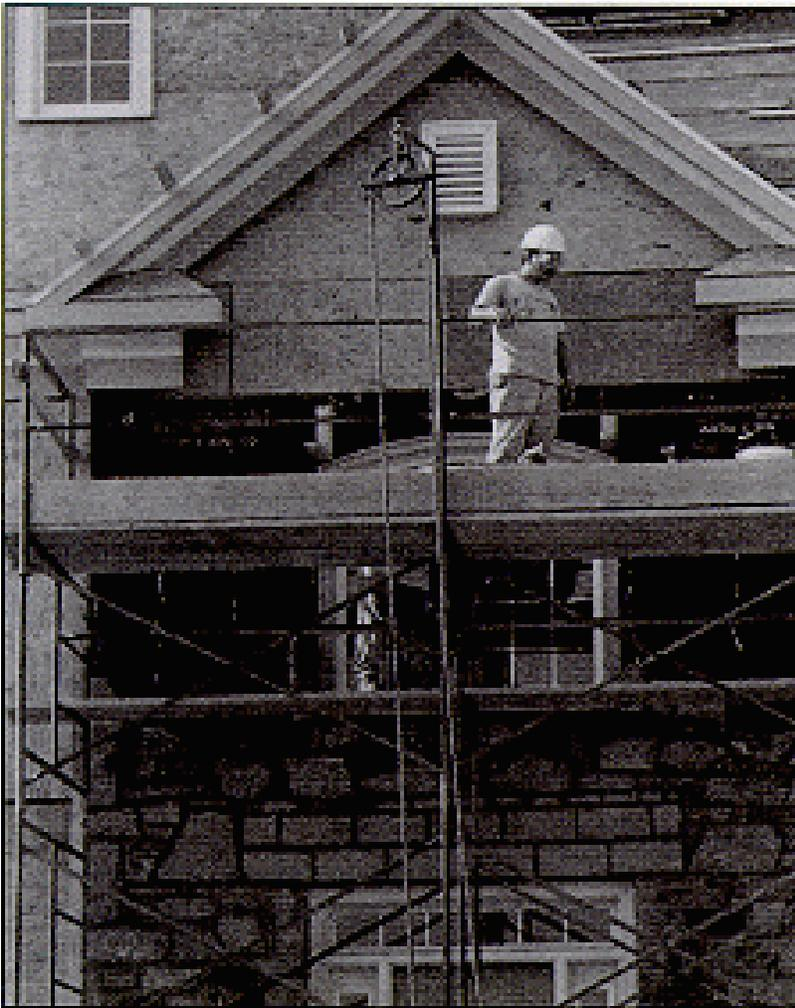
Workers are on a fabricated frame scaffold. There is ladder access to the top of the scaffold (out of view), guardrails and cross bracing are installed, and the planking is complete to prevent falls. The workers are also wearing hard hats and using eye protection.
