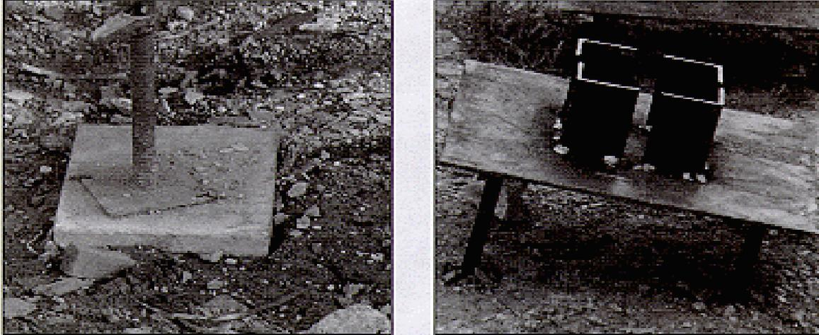
Stable footings/mud sills for this scaffold ensure the stability of the work platform. In this example (right), the siding contractor actually had the base plate manufactured to penetrate the ground while stabilizing the pump jack holes.
